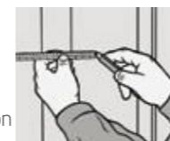
**UK:** Decide and mark the position of the frame in relation to the inner and outer wall.
