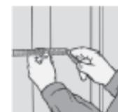
**UK:** Product to be offered into the structural opening. Always check aperture is clear of debris, check measurements of the opening match product for installation before offering product into structural opening.
