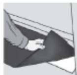
**UK:** If the base is of a concrete construction, a DPC must be placed under the full length of the threshold. Place door onto a bed of mastic.
