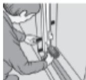
**UK:** Insert blocks to exactly fit at position of the frame fixing holes and locking points and fix with screws. On 2 leaf doors also in top and threshold. On doors over 2400mm in height or over 90 kg an extra bracket/fixing can be added on the hinge side at 200mm in from the corner.
