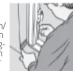
**UK:** Position frame in place according to predetermination position (5). Wedge at the bottom of each side (opposing wedges from inside and outside) so top can be adjusted without bottom moving.
